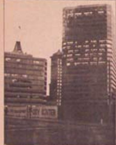
Completion of the Grove-Shafter Freeway is key to the completion of the City Center Project (bottom photo) and jobs for unemployed Oakland residents.
