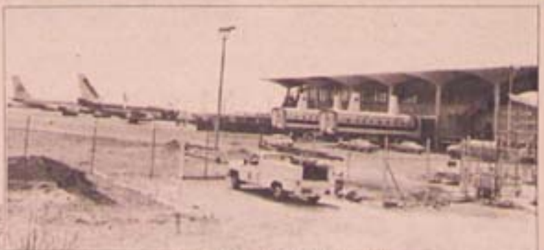
Construction site at Oakland Airport.
